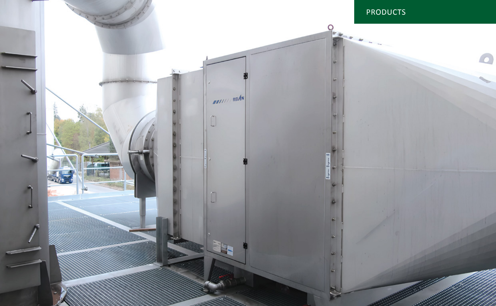
X-CYCLONE® RKM exhaust duct cleaner made from high-alloy stainless steel grade 1.4571 for use with very high exhaust airflow rates
