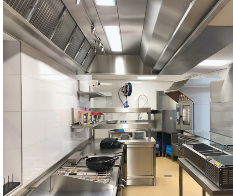
Induction hood with integrated fire-extinguishing system
