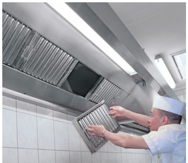
Stainless steel handles make it easier to handle the X-CYCLONE® separators in kitchen hoods.
