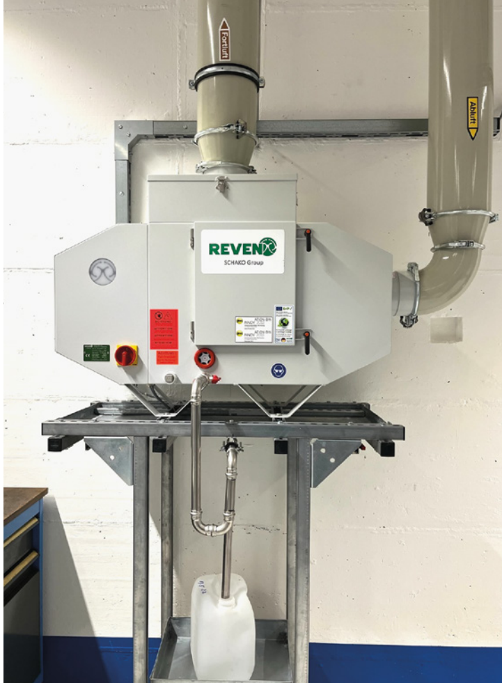
X-CYCLONE® C-XSC oil mist separator installed in a decentralised location
