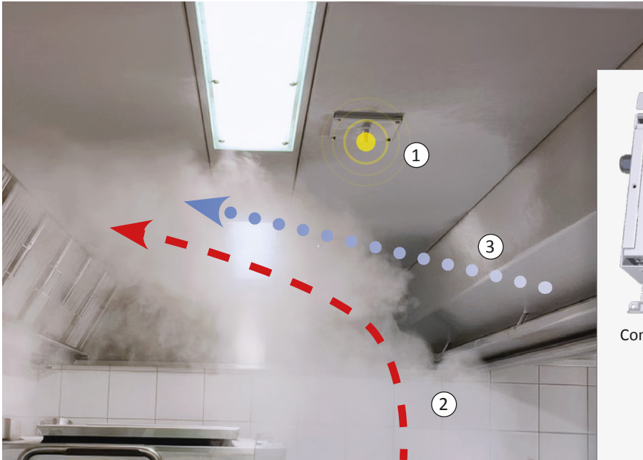
Use of the RSC control system in an induction hood
