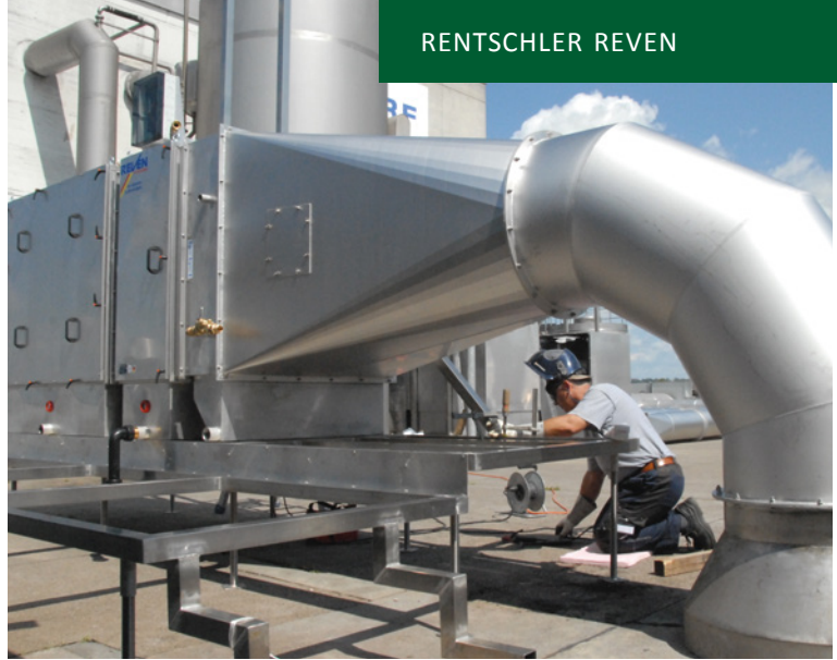
In-duct exhaust-air cleaner for food industry applications
