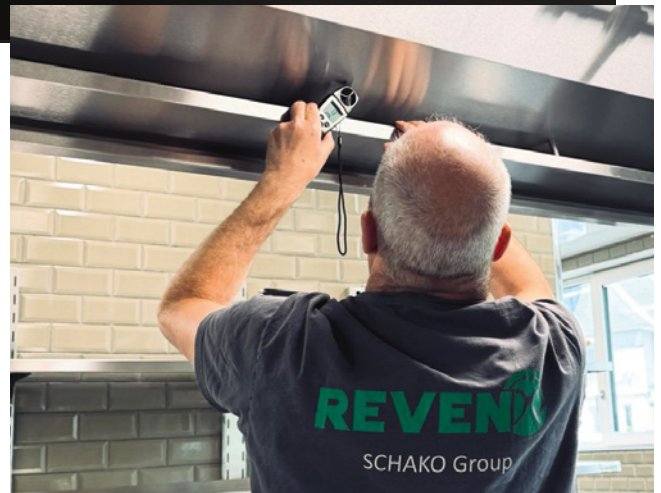
Final inspection of a fitted induction hood
