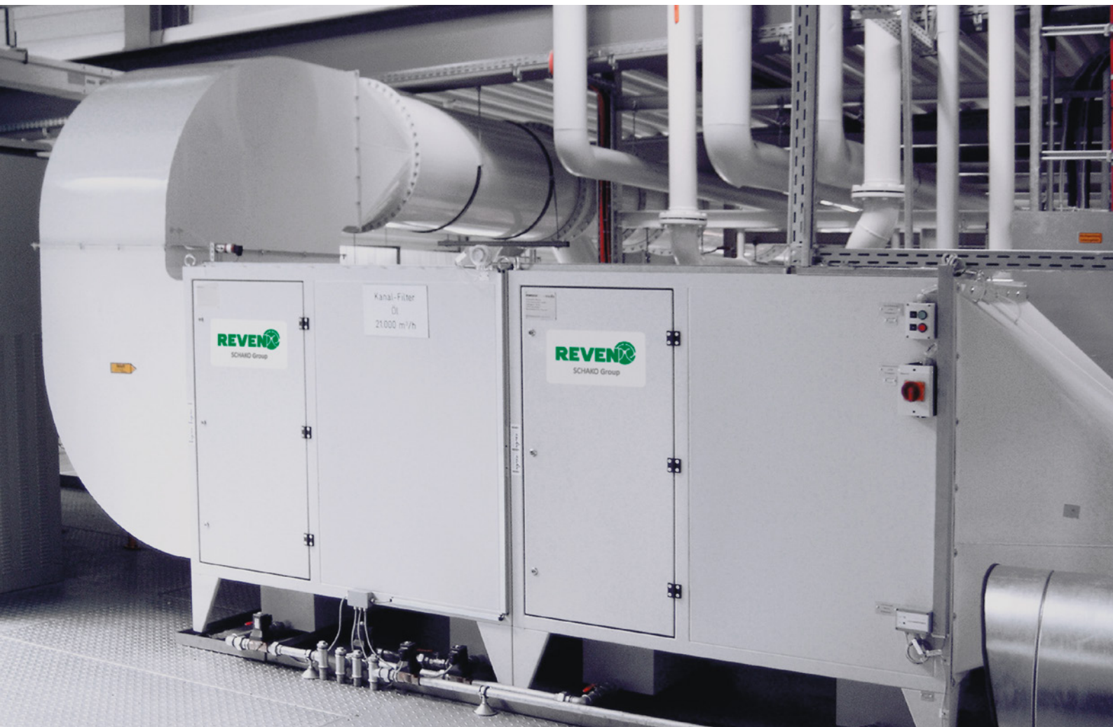
Two X-CYCLONE® RKM exhaust duct cleaners connected in series
