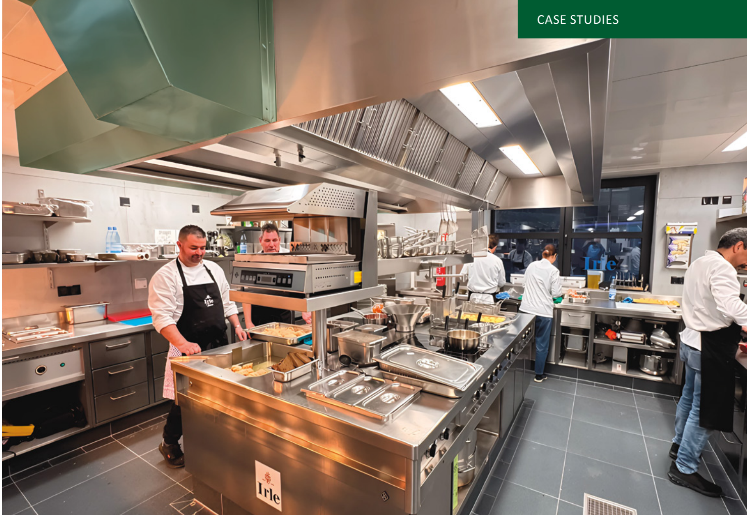
X-CYCLONE® EVN-M extraction hood, viewed from the front, with an air duct running around the left-hand side (shown in green)
