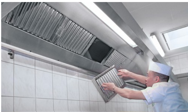
Removal of the X-CYCLONE® separators from an exhaust air hood.
