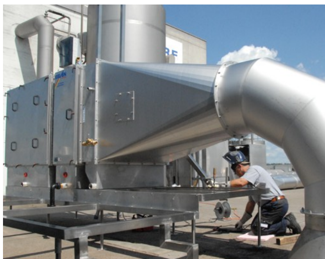
Installation of a REVEN duct separator in the food industry
