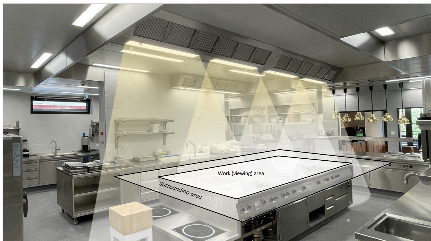
Fig.: When calculating for a work surface, the adjacent area, the surrounding area (a virtual border around the work surface), must be at least 50 cm. The illuminance for the work surface must be at least 500 lux and for the surrounding area 300 lux.
