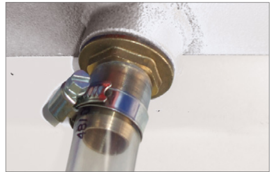
Fig.: Connection for oil return hose part no. 9090050004
