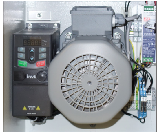
Fig.: Variable frequency drive installed in the motor cabinet (on the left)
