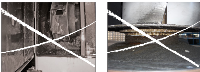
Fig.: View of the interior of a unit that was not maintained
