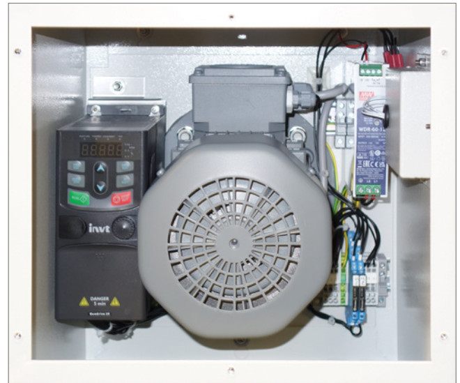
Fig.: Variable frequency drive installed in the motor cabinet (on the left)
